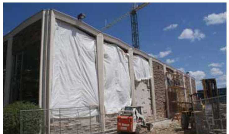
Insulation and stone work; exterior south wall
