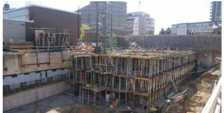
Underground garage taking shape
